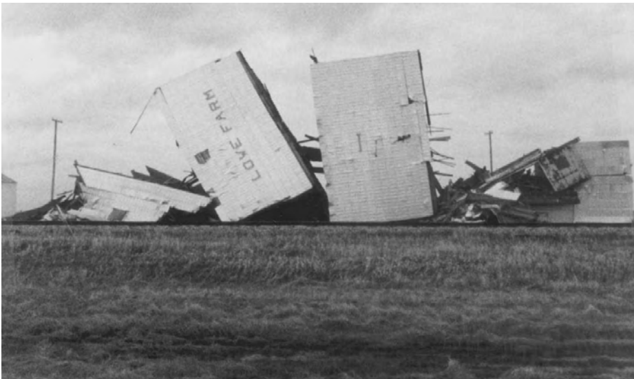
A UGG elevator is demolished in Lowe Farm, 1984.
