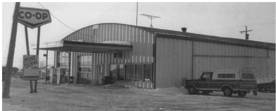
Lowe Farm Co-op Services Ltd. , 1980.
