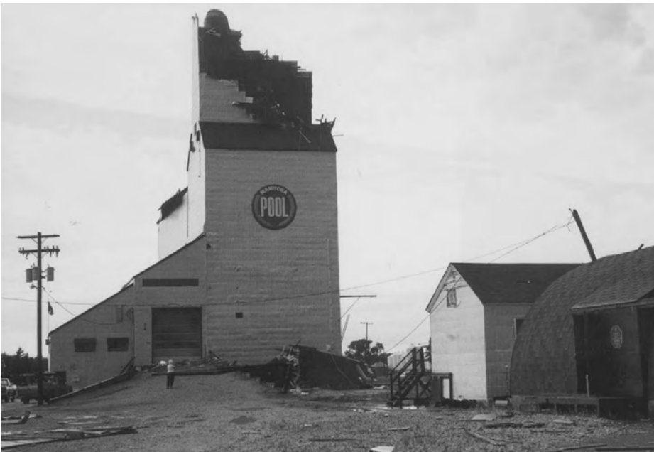
Lowe Farm Manitoba Pool Elevator damaged by wind on July 20, 1998.
