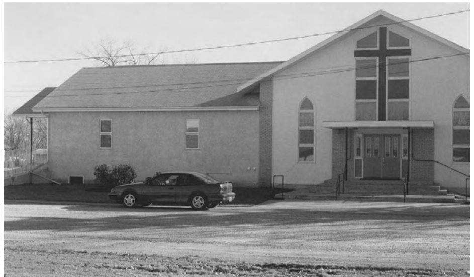
Completed church addition.
