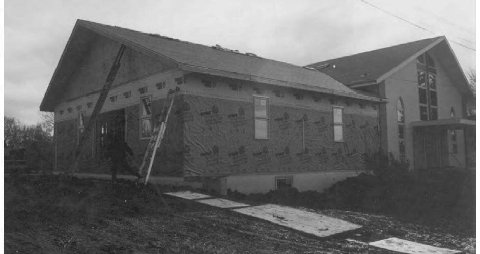
Church Addition in progress, 1994
