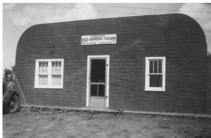
Egg grading station in Lowe Farm.
