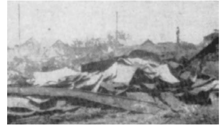
Aftermath of fire which swept through Lowe Farm's Main Street in 1921, destroying the Co-op, Reimer's I.H.C. shop and Johnson's' Garage.
