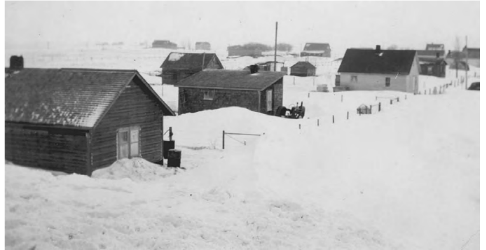
This Lowe Farm street won't be passable for some time.
