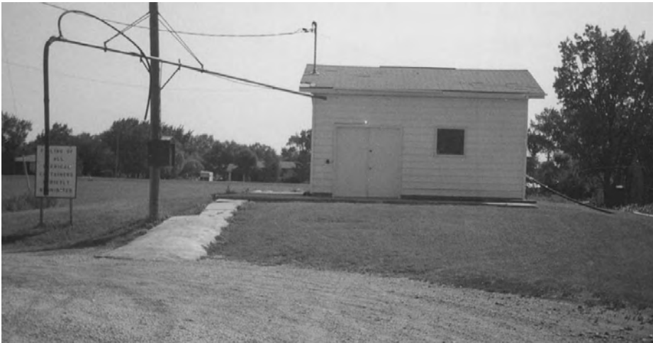
Pump house and water stand in Lowe Farm.
