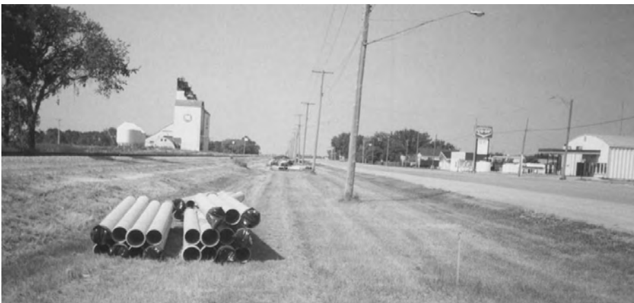
Pipe installation underway in 1998.
