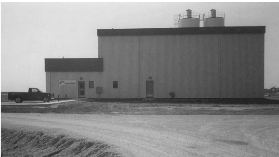
The new water station in Morris.
